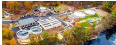
Wastewater Utility Management Newmarket, NH, Environmental Services
